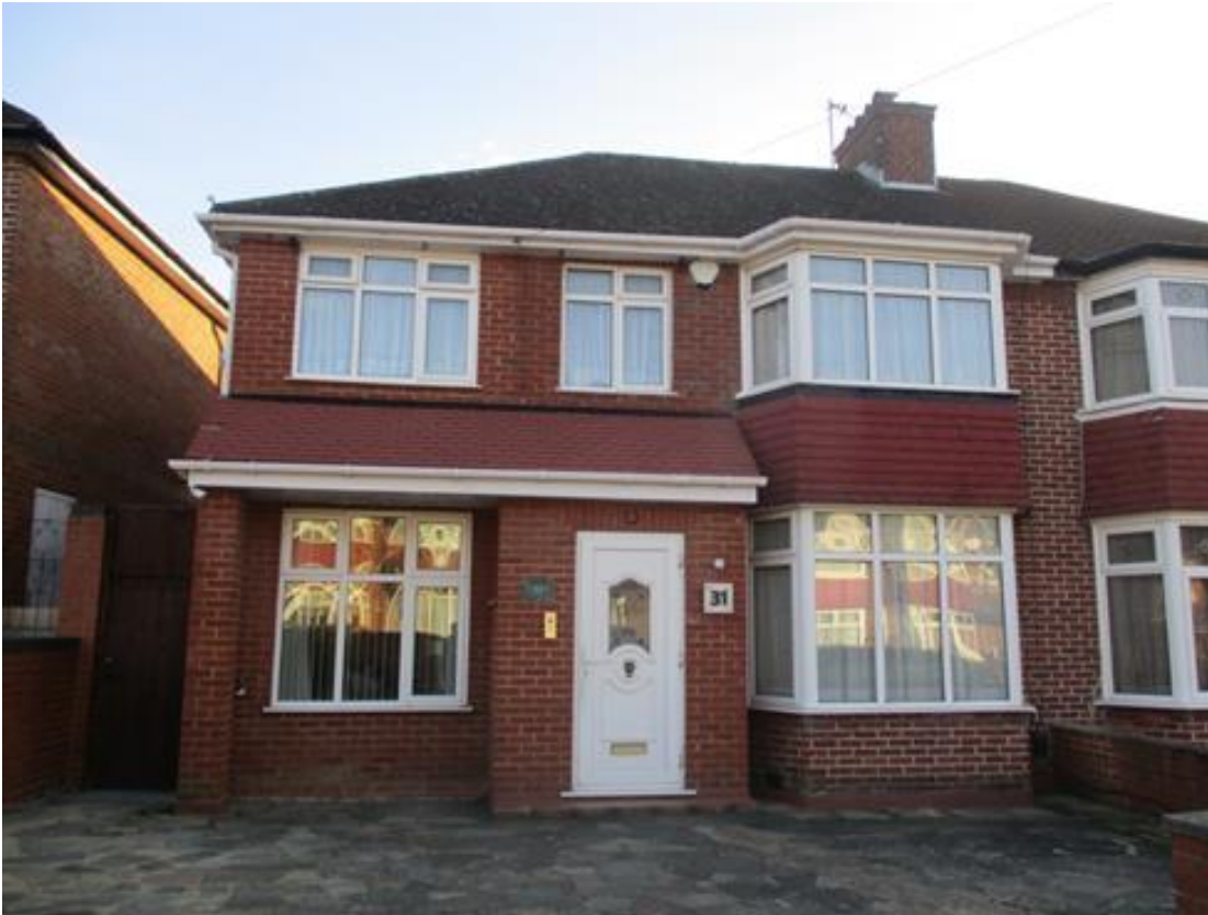
Front Elevation of no. 31 Coledale Drive
